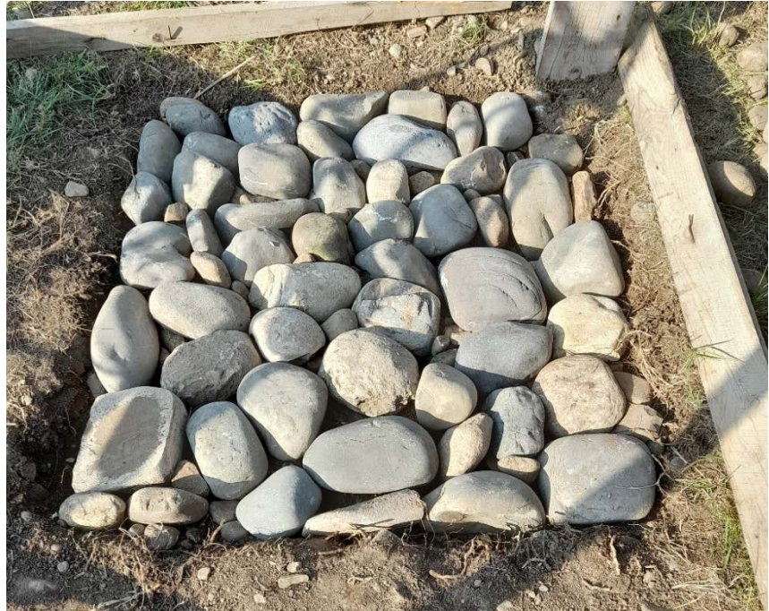
Pic.3. The foundation of the experimental oven.
