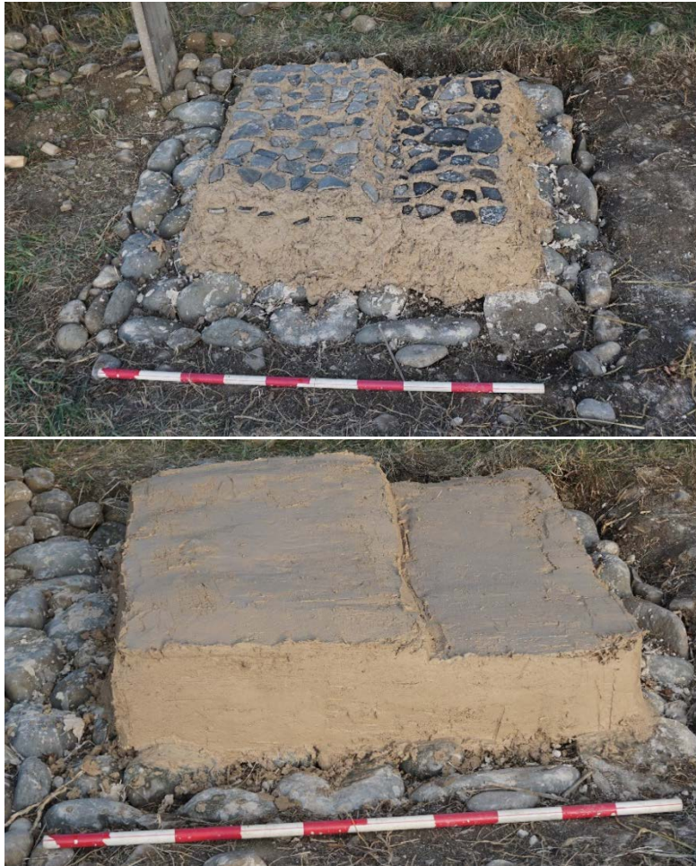
Pic.6. Preparing the baking and fire cameras of the oven.
