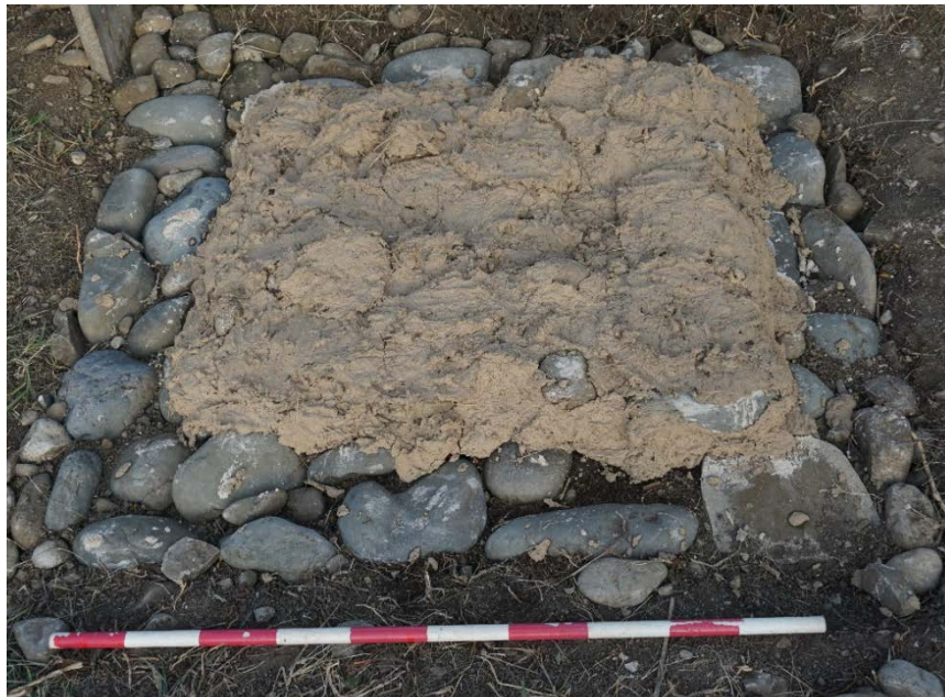
Pic.4. First layer of clay mass on the foundation.
